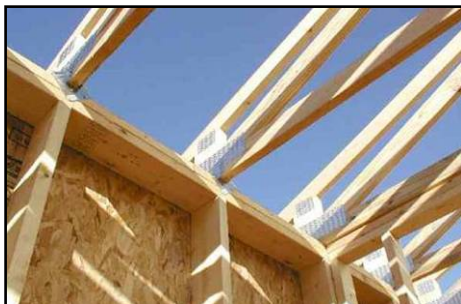
Raised heel roof trusses
